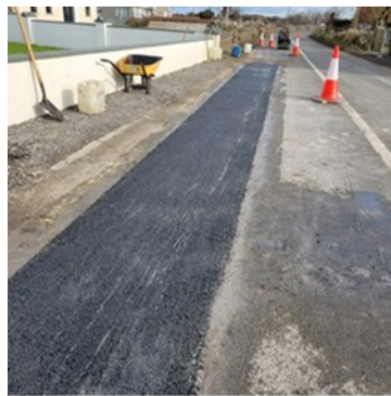
PERMANENT ROAD REINSTATEMENT FOLLOWING PIPING WORKS AT KILCONEIRON CHURCH, LOUGHREA, OPW MINOR WORKS PROJECT
