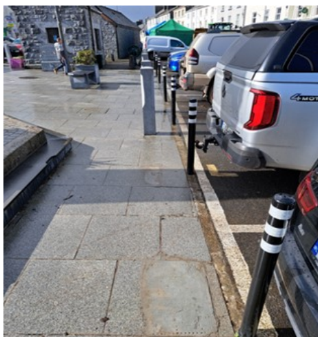
PLACEMENT OF FLEXIBLE BOLLARDS AT MAIN STREET, GORT TO PROTECT EXISTING STONE BOLLARDS
