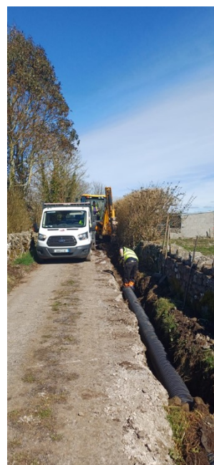
SURFACE WATER PIPING AT LIMEHILL, LOUGHREA IN PREPARATION FOR ROAD RESURFACING
