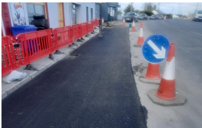
DRAINAGE WORKS IN KILKERRIN - PIPELINE AND GULLIES INSTALLED WITH PARKING AREA RE-GRADED TO ELIMINATE FLOODING.
